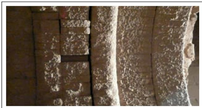
**Figure 2.** Lining damage after 3 months in operation.
