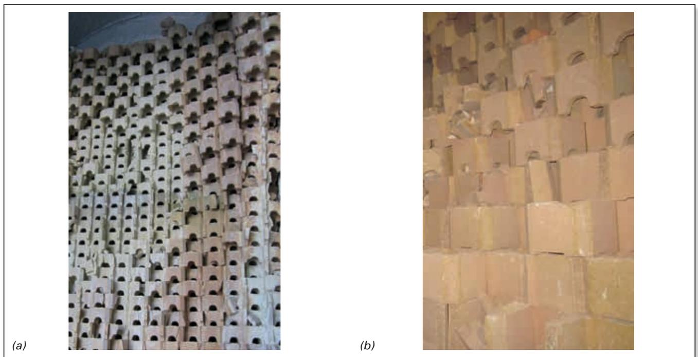
**Figure 8.** Checker work after 8 years in operation. (a) ANKER DG1 in the regenerator upper region and (b) RUBINAL EZ in the condensation zone.
