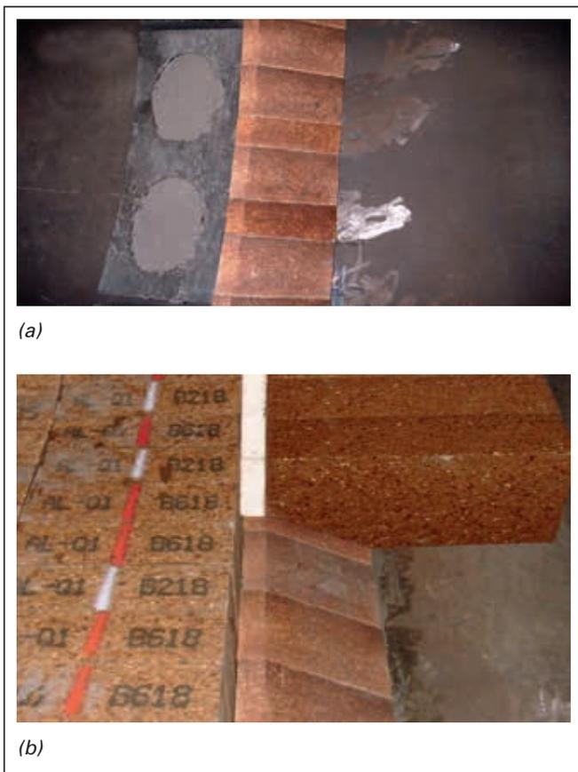
**Figure 4.** Installation of the (a) first ring of skew bricks and (b) second Thrust Lock System shape.
