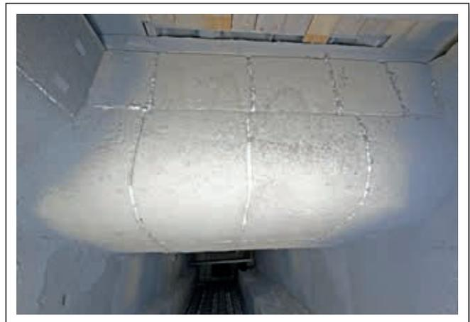
**Figure 4.** Bullnose after joint maintenance showing the same area as in Figure 3 after a further 8 months of operation, no significant change can be identified. After 15 months in operation, the mix remains in the cooler without any further repair required.
