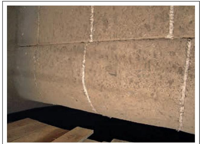
**Figure 3.** Bullnose lined with CARSIT SOL M10G-6 after joint maintenance. After 7 months no wear was identified.
