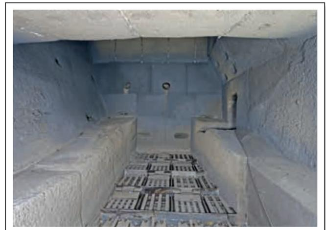
**Figure 7.** Clinker bed with CARSIT SOL S30-6 after 15 months in operation.
