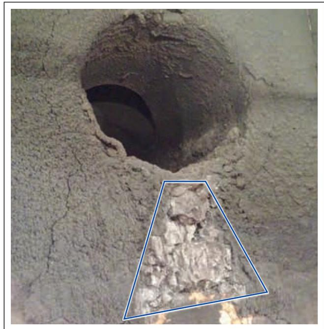
**Figure 8.** Evaluation of severe localized corrosion of the lining below combustion chamber of a pelletizing furnace after 9 months of operation. The highlighted region requires an individual refractory design and material selection.
