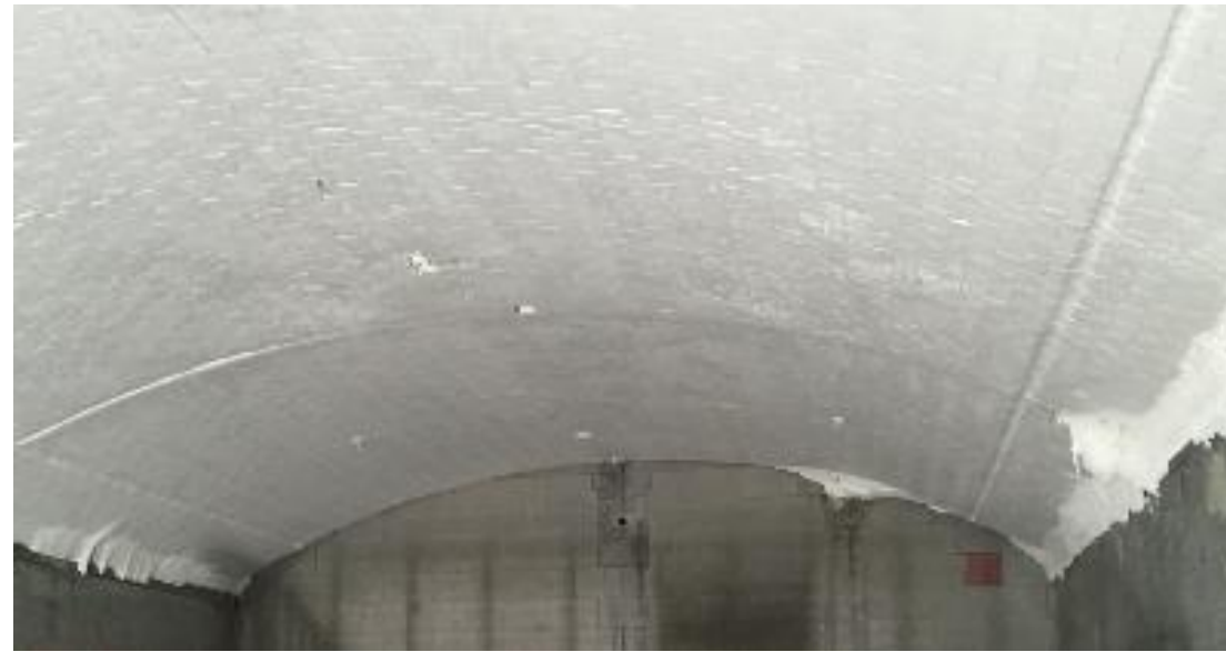
Stella GNL after 10years in an oxyfuel furnace
