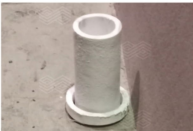
Figure 3. Starter tube and starter ring installed in a tundish.
