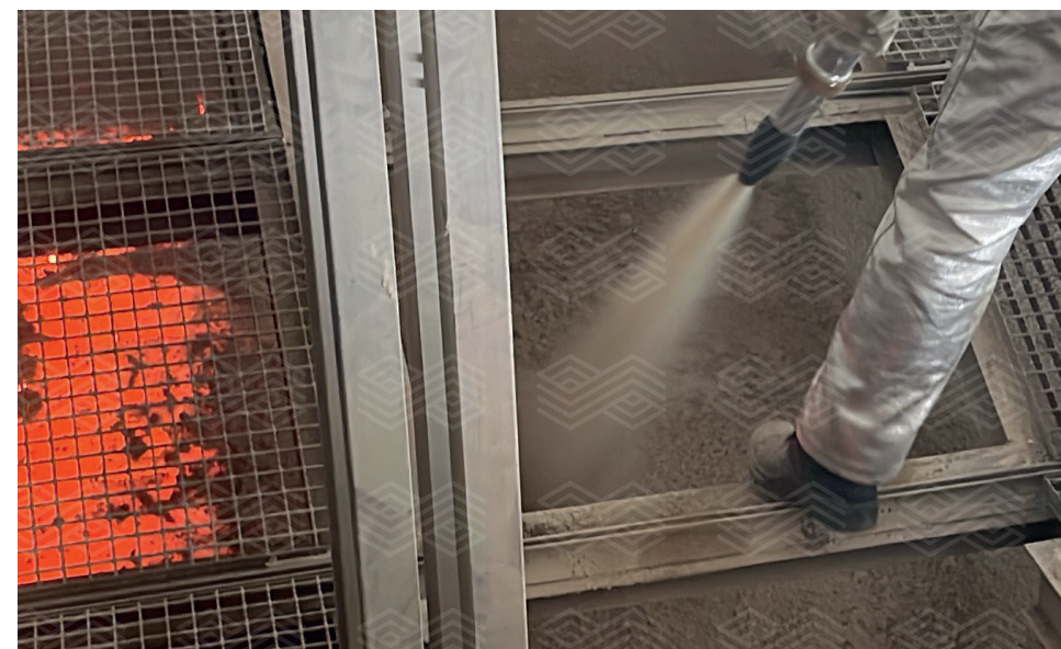
Drygunning on a crown
